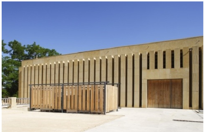
Gilles Perraudin's Wine cellar in massive stone for the Solan Monastery in southern France.
